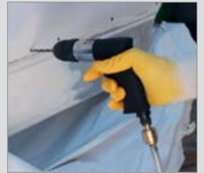
Drilling – in wood, metal or concrete
