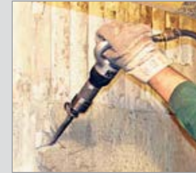
Effortless removal of plaster and tiles
