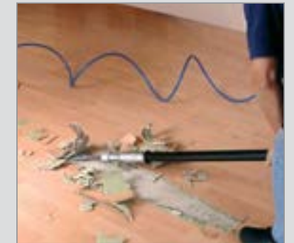
Floor coverings stripped with ease
